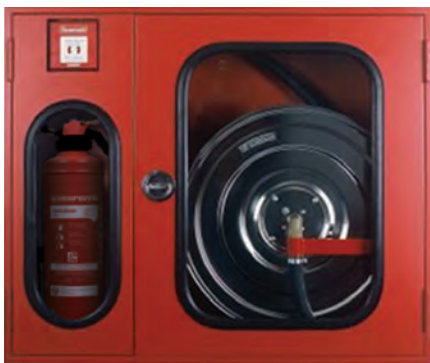
Wall Hydrants & Hosereels
